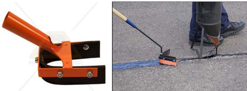
Figure 2.5: Typical flat finishing techniques ( http://www.battseal.com/residential.php )
