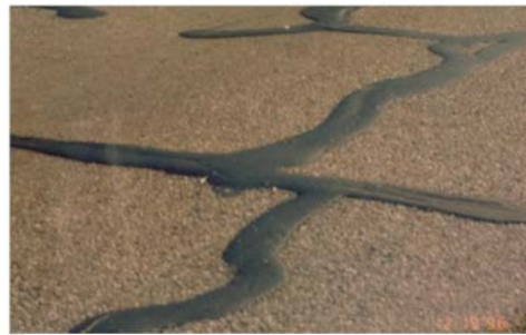
(b) Raised and Bumpy Sealing
