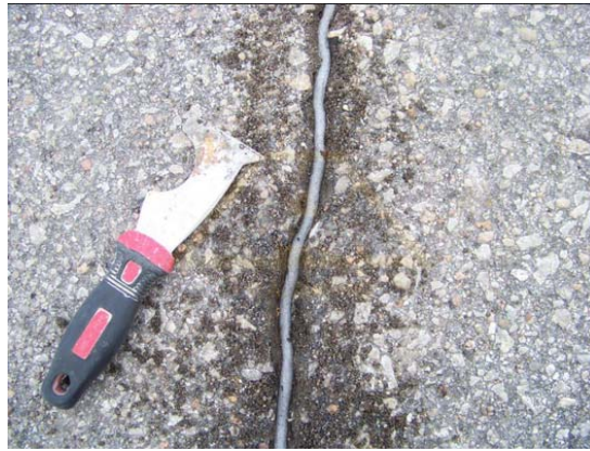
Figure 2.3: Application of Backer Rod
