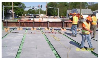
Figure 2.5 NYSDOT Bulb-Tee Girders with Shear Pocket Ready for UHPC Pour
