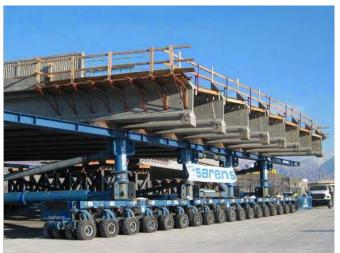
Figure 2.16 Sam White Bridge in Utah Being Moved into Place Using SPMTs
