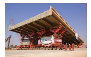
Figure 2.13 Bridge Span Being Moved with SPMTs
