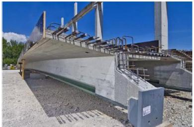
Figure 2.18 Prefabricated VFT Girder
