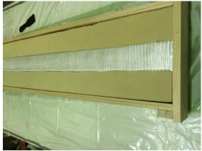
(c) Installing Foam and Laying Shear Fiber
