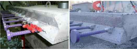
Figure 2.9 Headed studs Extending out of Deck Panel
