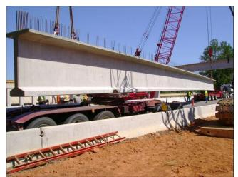
Figure 2.11 Moving Prefabricated Bridge Element into Place at Construction Site
