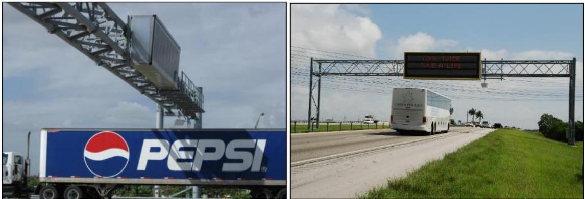
Figure 1.1 VMS structures on Florida's Turnpike (a) side elevation (b) front elevation
