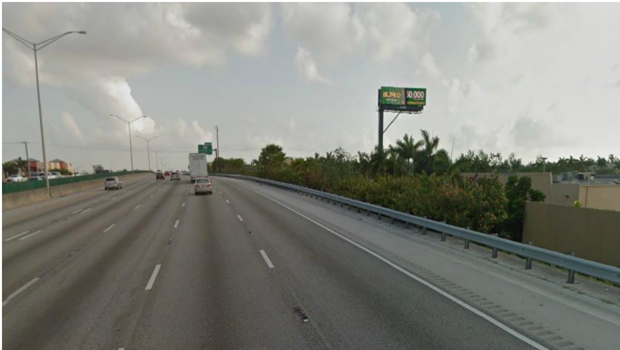
Figure 3.13: Location ID 9 on I-95 NB in Hallandale Beach
