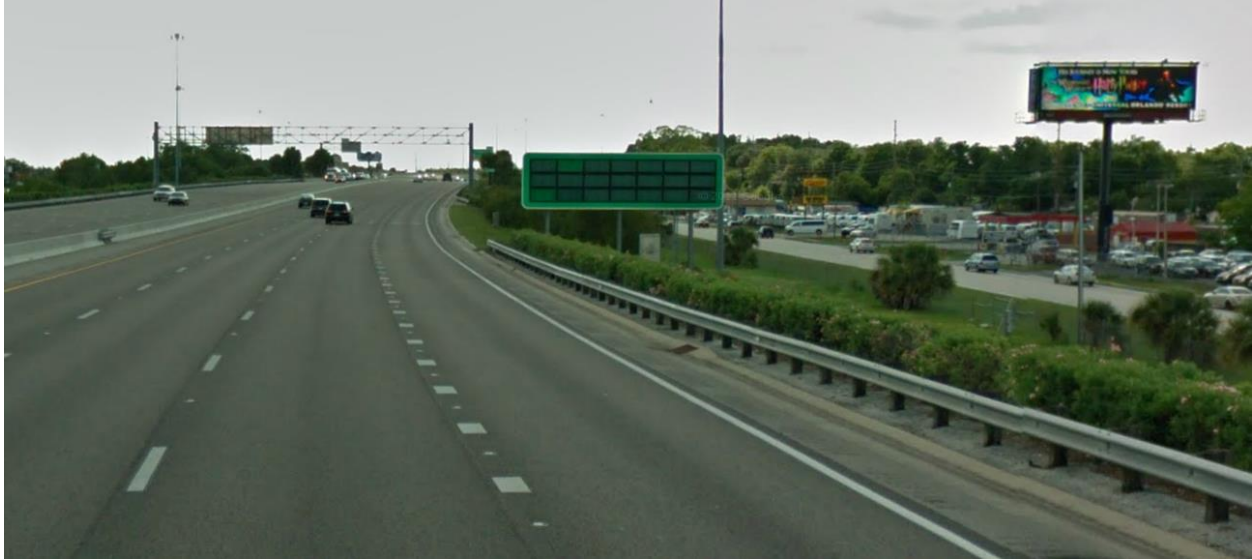
Figure 3.16: Location ID 18 on SR 528 WB in Orlando
