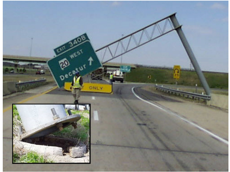
Anchor bolt sign failure.
