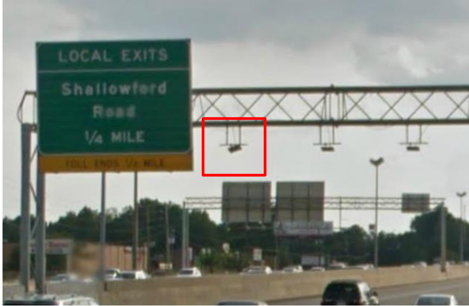
Figure 60: Misaligned General Purpose Detector
