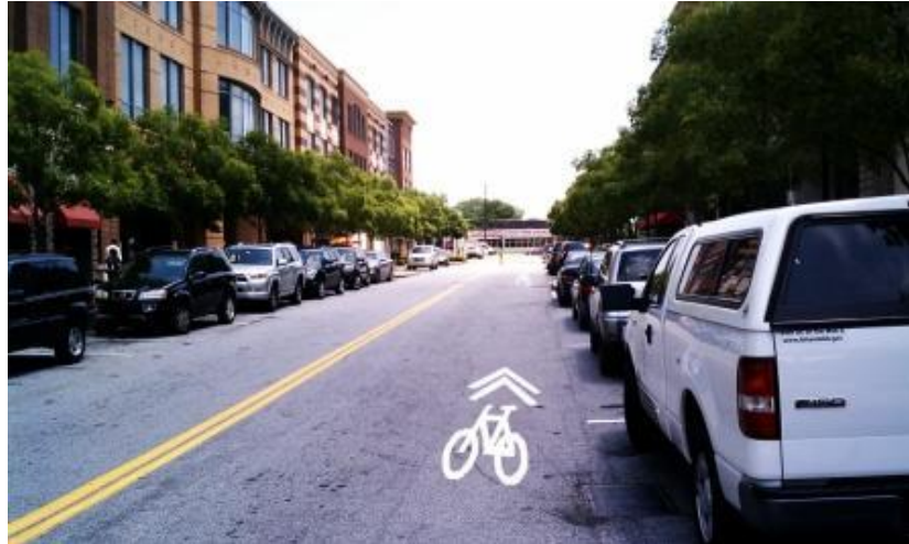
Figure 6: Sharrow Pavement Marking
