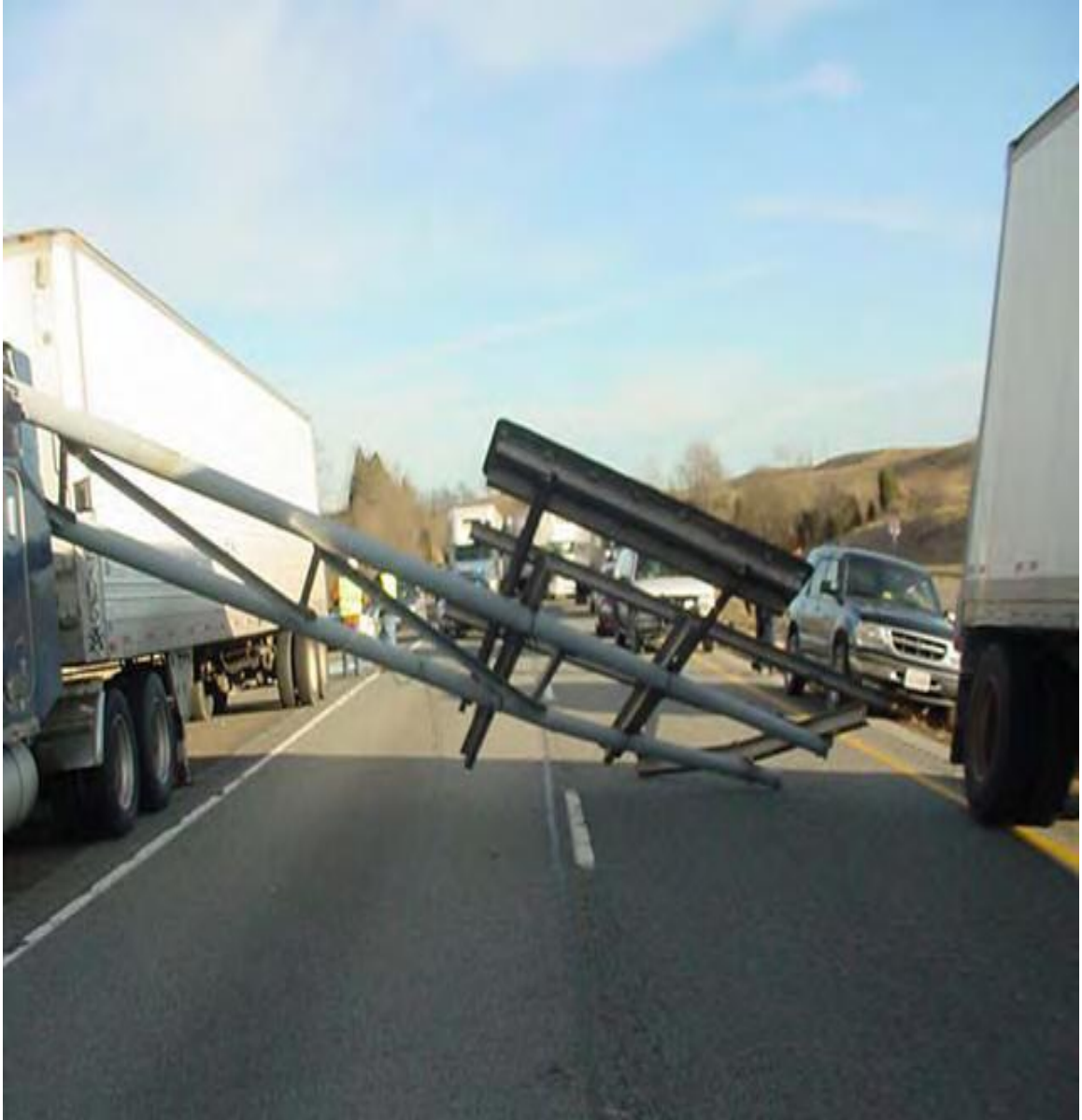
Figure 2.14 A Failed Cantilever Sign Structure [40]
