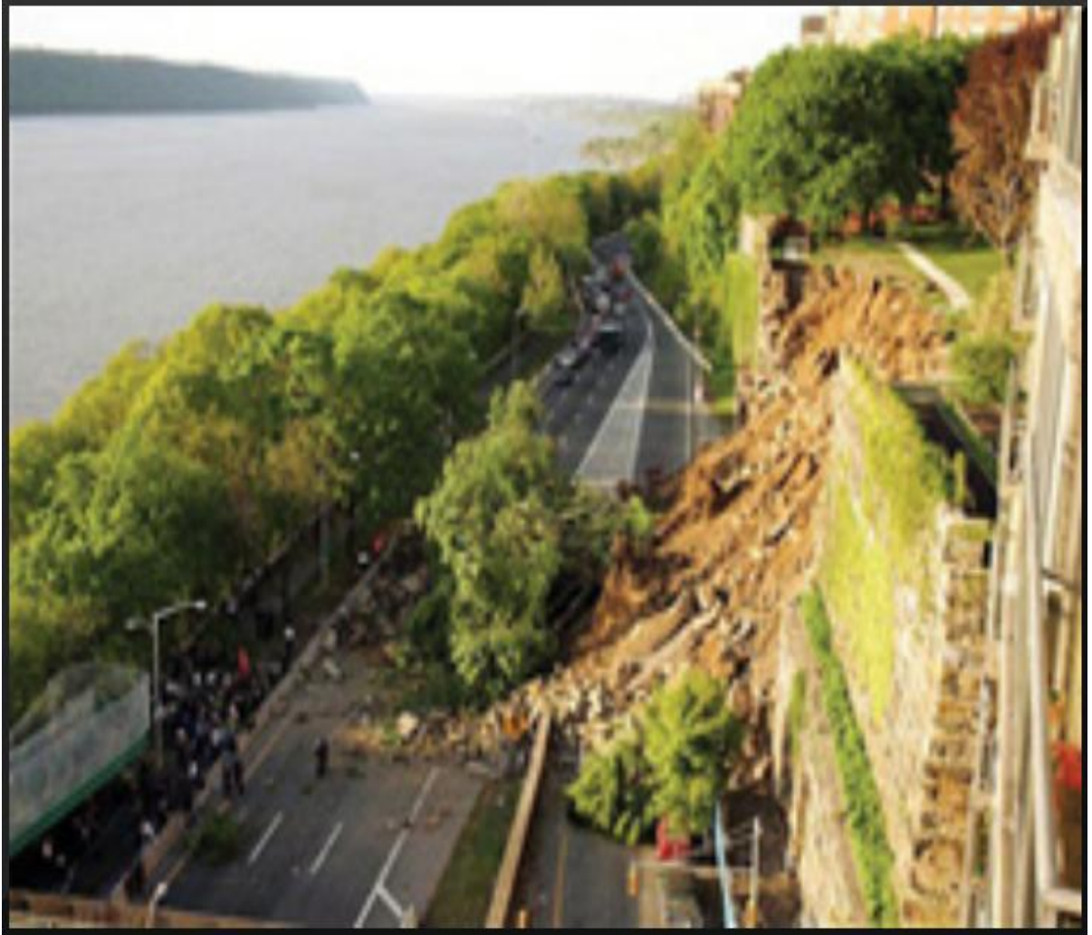
Figure 2.15 Failed Earth Retaining Structure along Riverside Drive near Manhattan in New York [37]
