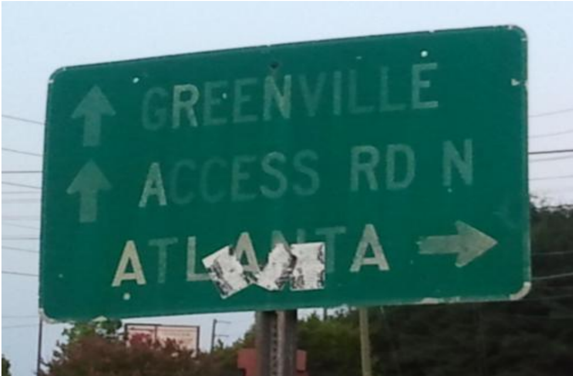
Figure 2.13 Example of a Failing Road Sign
