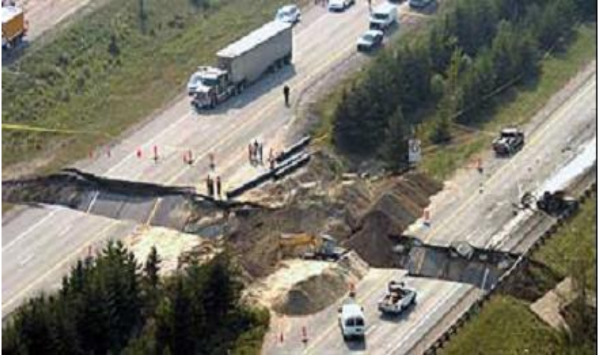
Figure 2.12 Highway-40 Failure in 2005 between Montreal and Quebec City [46]
