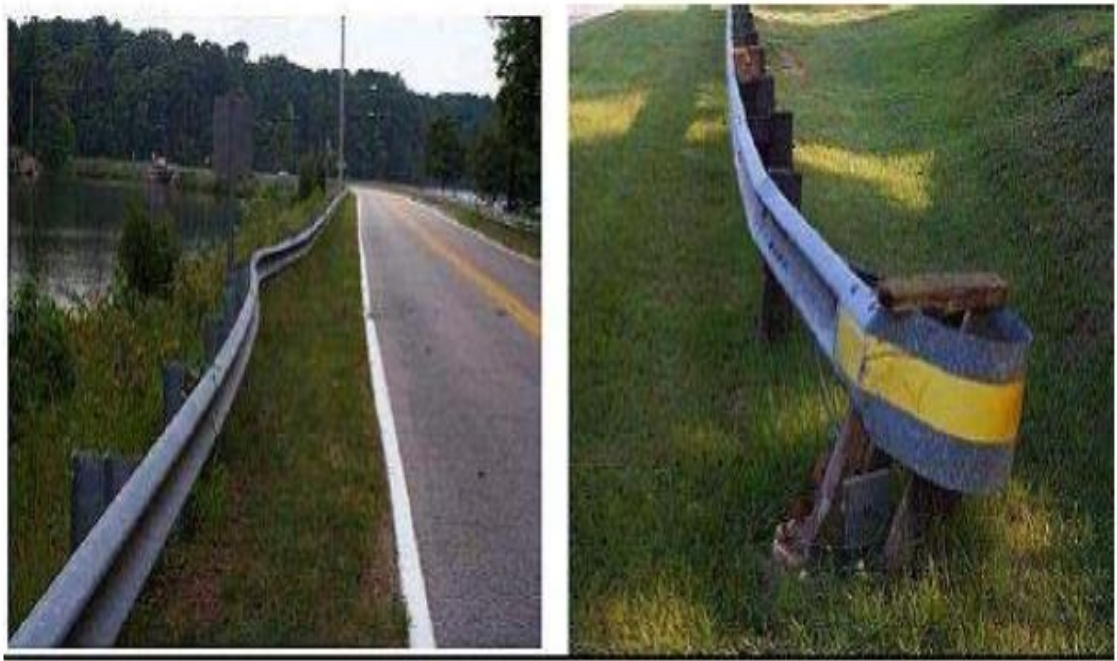
Figure 2.16 Damaged Guardrails [50]
