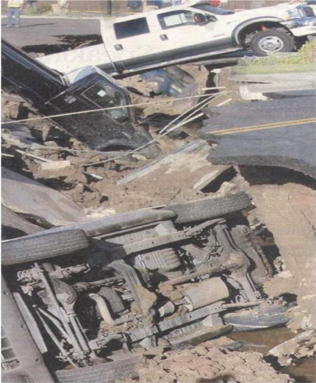
Figure 2.10 Bakersfield, California Sinkhole [46]
