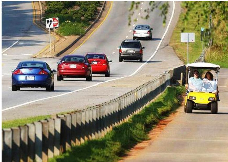
**Figure 10. Peachtree City Electric Cart on Separated Path (Hollis, 2008)**
